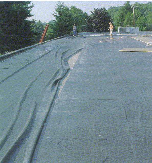
EPDM roof sheeting installation
